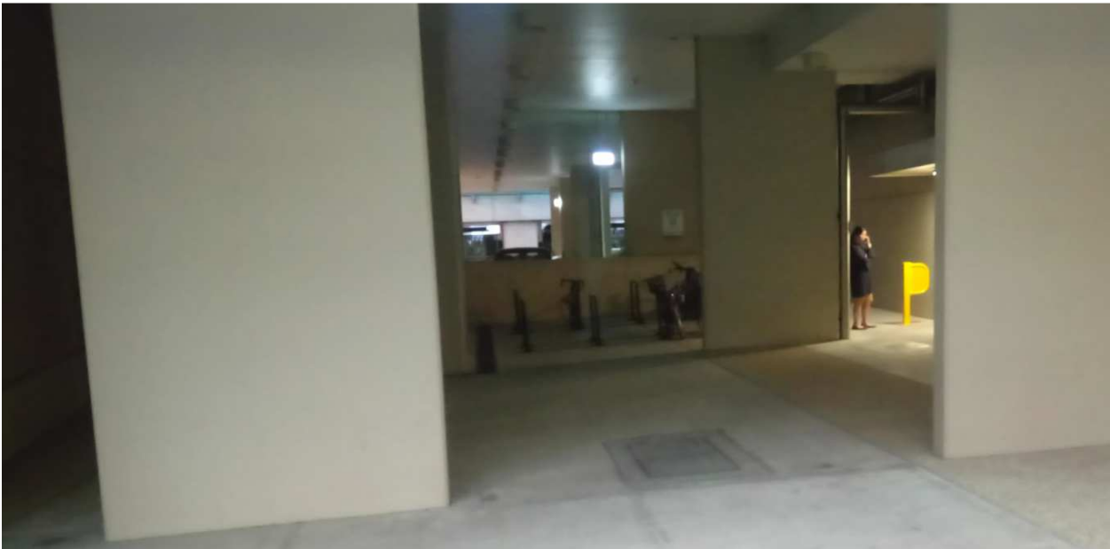
Figure 2 - Bike parking but with poor passive surveillance
