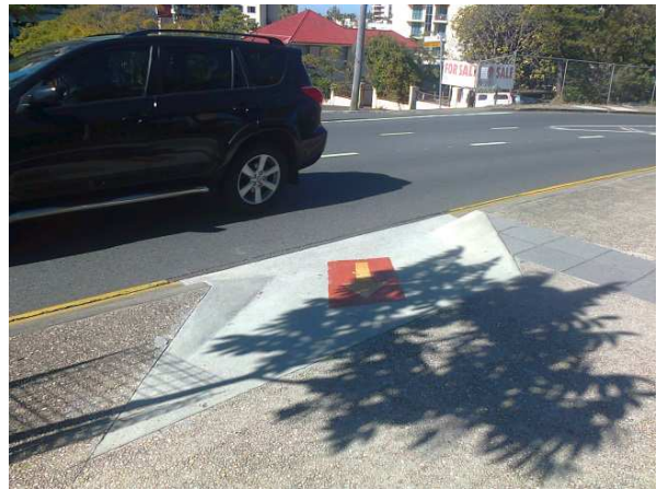
Figure 4 – Example - Existing bike kerb ramp Deakin St, Kangaroo Point
