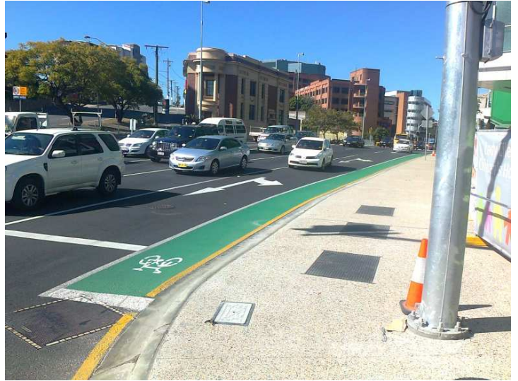
Figure 2 – Stanley St bike lane at the intersection with Graham St. Bicycle press button and kerb ramp required
