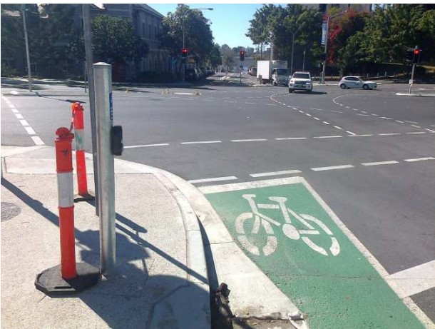
Figure 3 – Existing Bicycle press button, Graham St bike lane at the intersection with Stanley St
